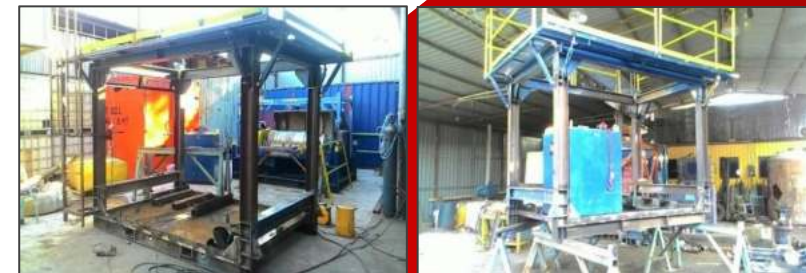
Refurbishment / modification - Centrifuge Skid
