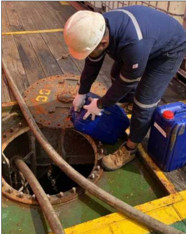
FLUSH LINE ACTIVITY CONDUCTED BY VESSEL MASTER
