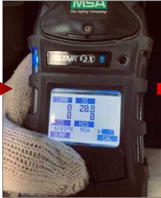
AGT CONDUCTED GAS TESTING BEFORE ENTERING MANHOLE
